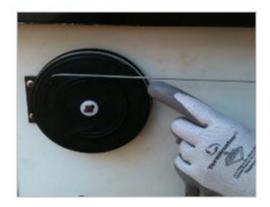
*NOTE*: White dot is reference to cable breakover on to flat channel, for optimum reaction and tension on door in closed position. ADDITIONAL WRAPS BEYOND THIS POINT WILL DIMENISH REACTION AND TENSION.
