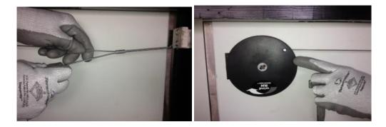
**4)** Holding each cable, with each hand, pull line off spirator towards fastening point. At same time pull loose end toward spirator until **cable** is **even** with **white dot** on spirator.
